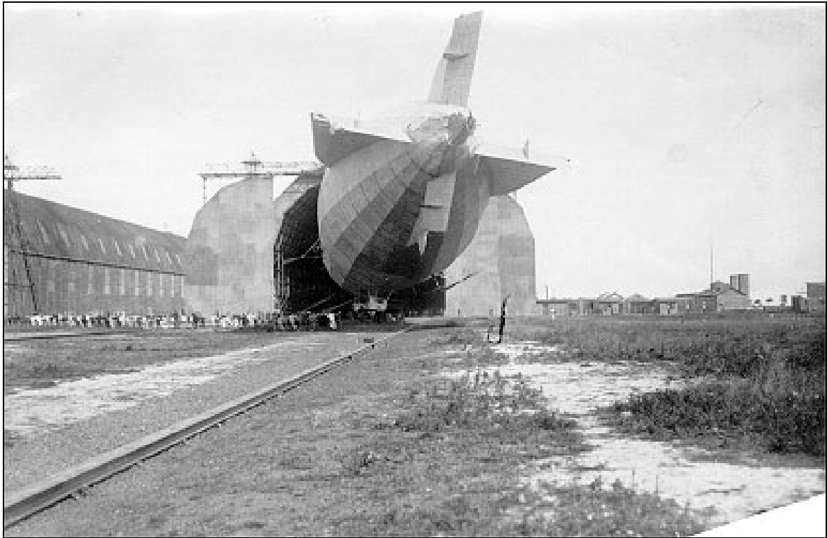
Zeppelin L-11 being taken out of her shed at Nordholz. Note the damage to her stern.
